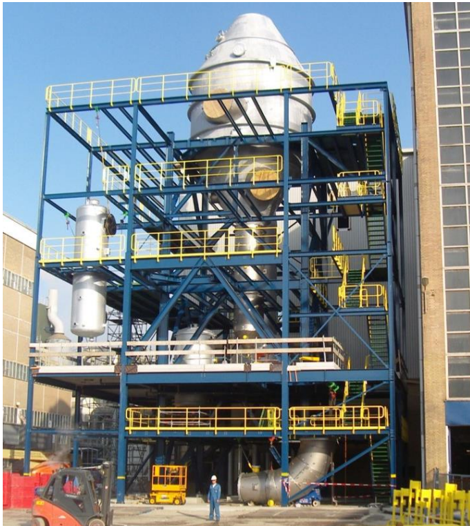
Figure A1: Current heat pump (MVR) in Delfzijl
