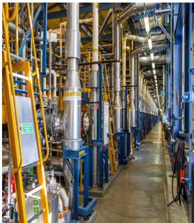
Figure 7.3: Electrolyzers for chlor-alkali production in Rotterdam
